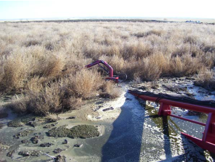
Submersed Slurry Gate in Heavily Overgrown Lagoon
